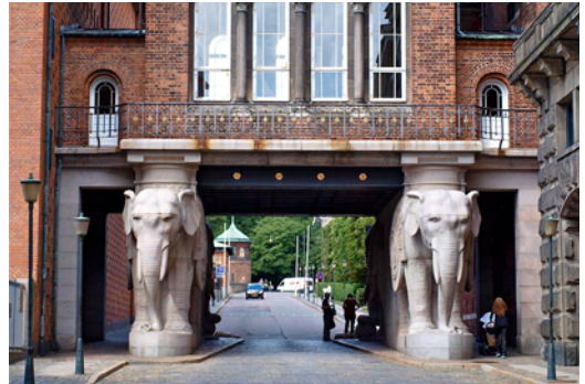
Figure 7 – The entrance to the Carlsberg Brewery area between the foundations of the "Elephant tower", built by architect Vilhelm Dahlerup, 1901
