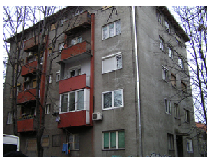
Figure 11a – View of the buildings type 2 (in the streets Vojvode Micka) before the refurbishment (source: Krstic-Furundzic A., 2012)
