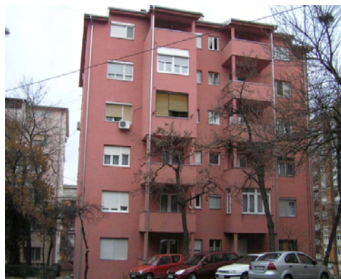
Figure 11b – View of the buildings type 2 (in the streets Vojvode Micka) after the refurbishment (source: Krstic-Furundzic A., 2012)
