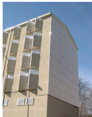
Figure 14 – Rehabilitated building – North and East façades
